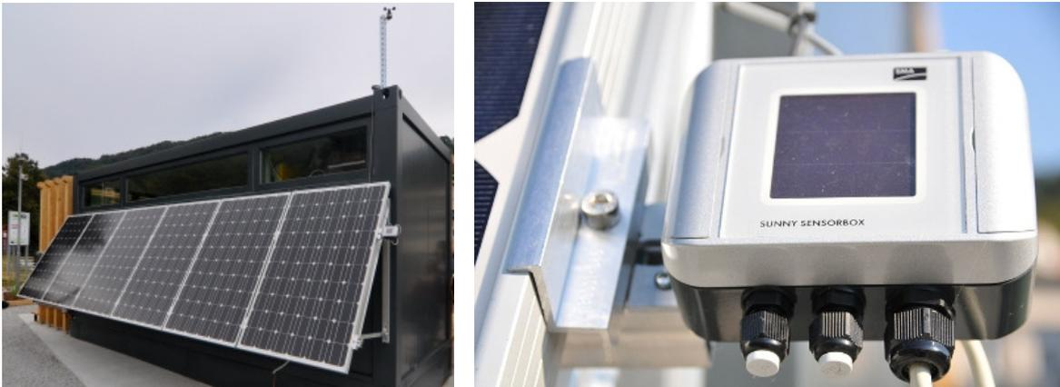
Fig. 6. OLEA off grid system (left) and its radiation sensor (right)
